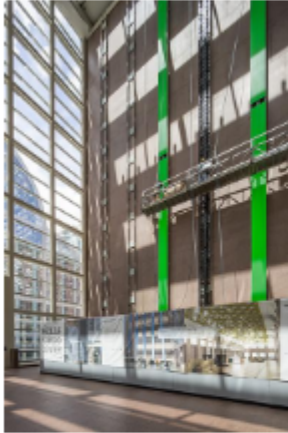
Installing the 8-story LED columns
